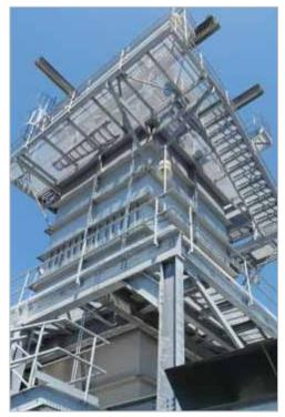
VG Engineering designs and supplies advanced custom gas turbine intake, vent and exhaust silencer systems to mitigate power generation and compressor station noise pollution. Our experienced engineers fully validated designs using in-house data together with CFD and FEA modelling to ensure acoustical, flow, thermal and structural requirements are met.
